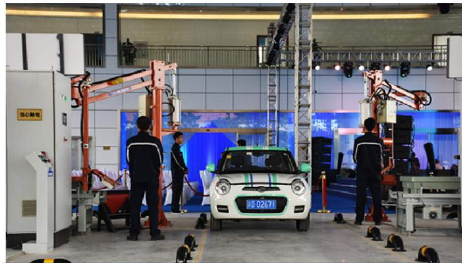
Battery swap station
